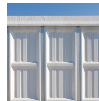
System cassette wall elements of hard-PVC
