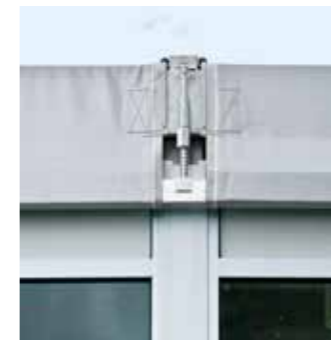
Spindle-fix roof tensioning
