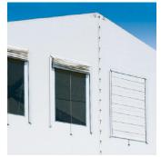
Cord-guided gable vent with folding cover (patented design), gable cover with plug fastening
